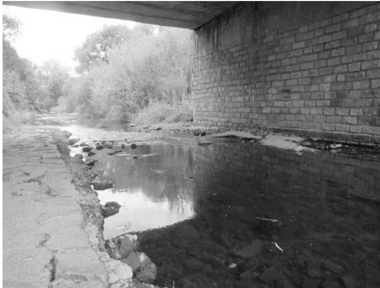
Fig. 6-3. Corridor for otter movement under bridge in Czech. It reduce otter casualties by vehicle.
